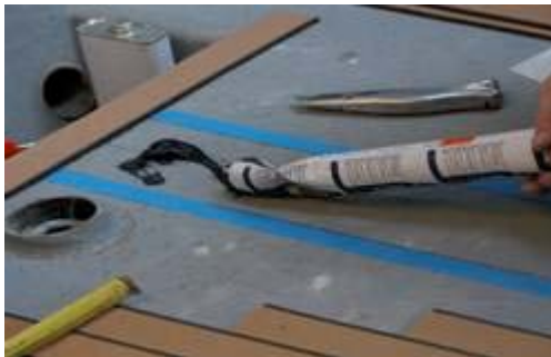
King Plank taped and adhesive applied
