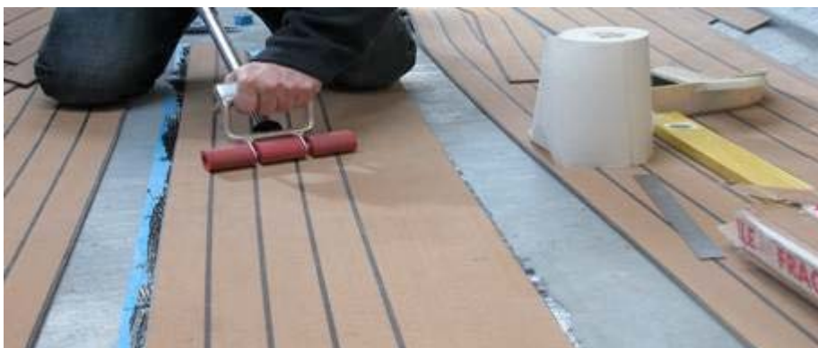
Four lengths of WDK100 joined together with Stelmax and laid in one operation. Once in place this is rolled to ensure no air bubbles and good seating on to the adhesive.
