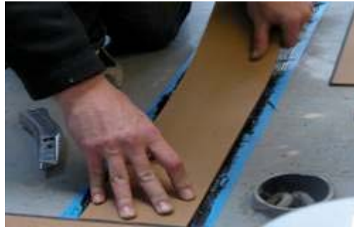
King Plank being laid
