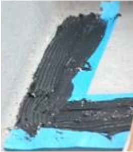
Margin taped and Adhesive applied.
